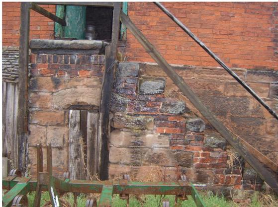
Picture B.12 External stairs are an example of a feature which should be identified and retained as part of any refurbishment
