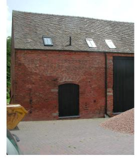
Picture B.8 A further example of a refurbishment which maintains an unbroken roofline
