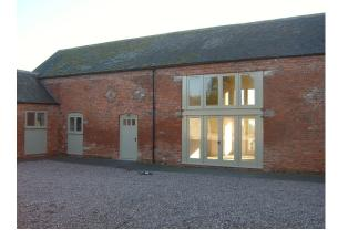
Picture B.3 Example of utilising existing openings to maximise natural, internal light
