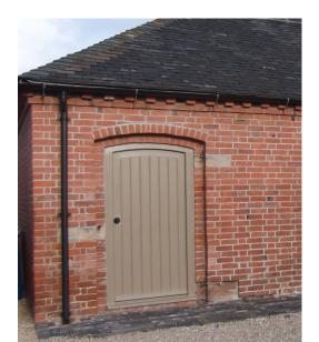
Picture B.9 A further example of repaired 'rise and fall' guttering
