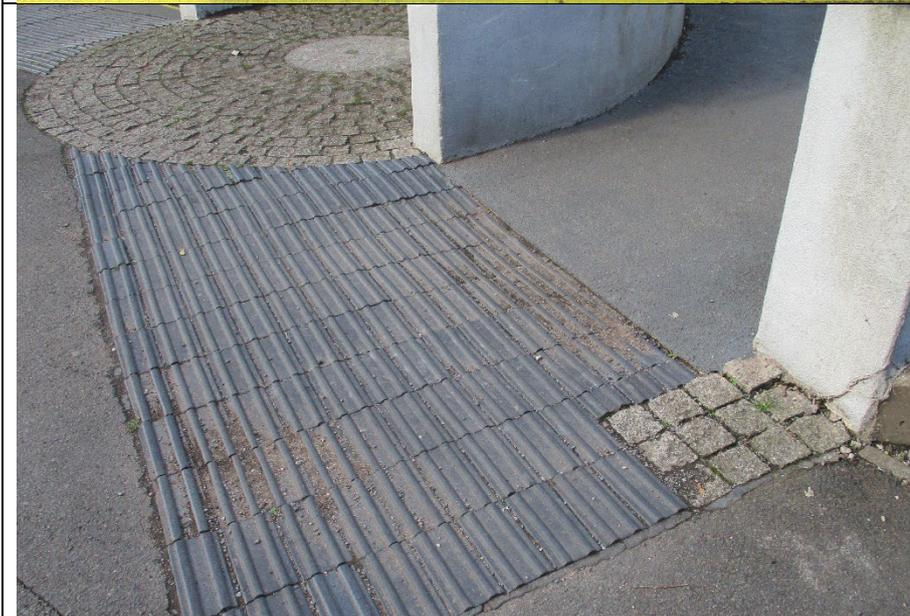
Foot of the curved pedestrian ramp showing incorrect use of tactiles. There should be no tactile warning to a ramp as it is not a hazard,
