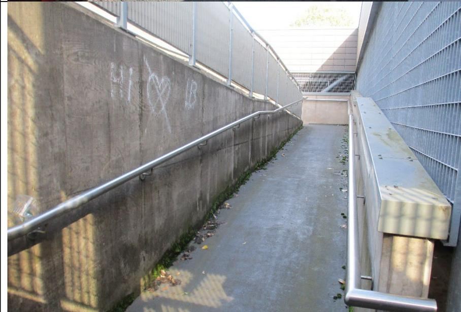
Lombard Car Park lower level access ramp which is long and steep but does have level landings (it is preferred that the landings contrast with the going of the ramp).
