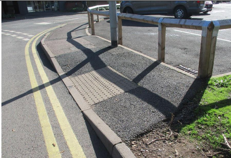
The nearest dropped kerb access showing a steep slope and insufficient level landing to allow a wheelchair to turn safely
