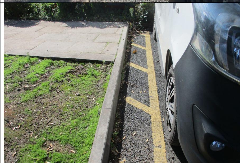
The side of the bay showing insufficient space for a passenger to transfer and no dropped kerb access
