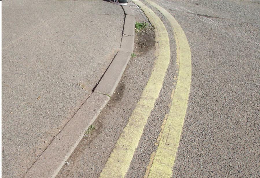
The poor dropped kerb, with an upstand and without tactiles, in the walkway to Market Street
