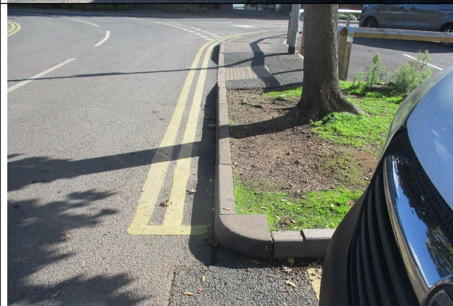
The ground alongside the bays showing no dropped kerb access and an uneven, muddy verge
