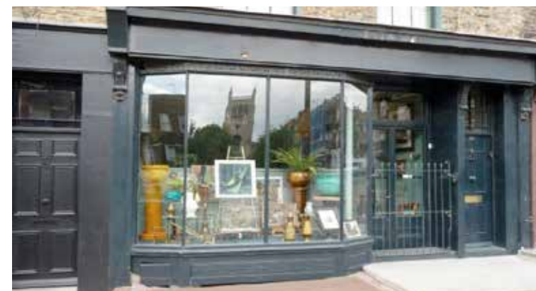
Figure CC.43. Painted timber shop front
