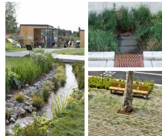
Figure CC.22. Example of surface run-off treatment
