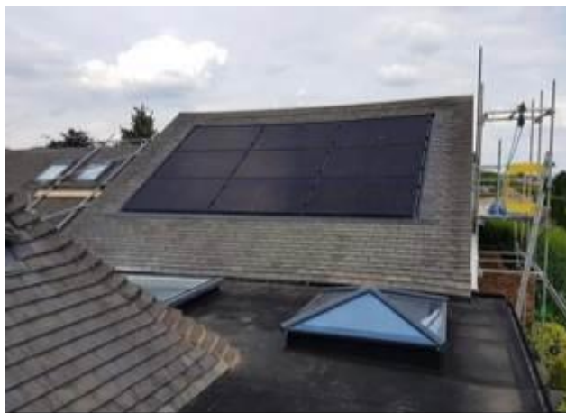
Solar panels sitting flush to the roofline on a property in Shenstone
