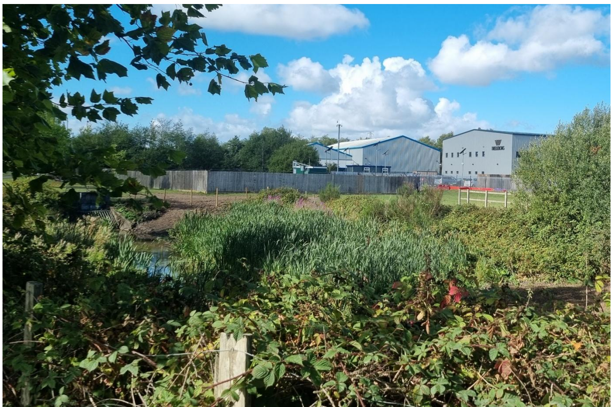
Figure 4.16: Attenuation pond on the edge of Burntwood Business Park
