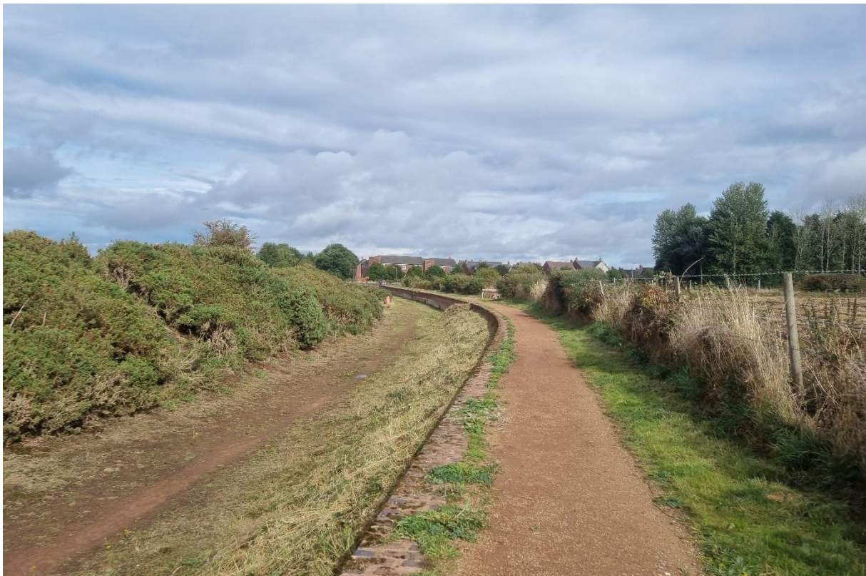
Figure 4.8: Restored section of the Lichfield Canal at Fosseway Heath, now forms part of the Heritage Towpath Trail
