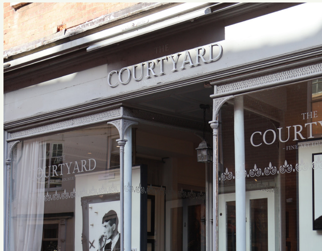
Clockwise from left: An excellent late 19th century shopfront on an 18th century building, on Market Square, featuring slender cast iron mullions and ventilation grills, a low stall riser base and a canopy awning with stay rods; Victorian shopfront; Well-preserved Georgian ground-floor bowed windows in Lichfield featuring convex cornicing, long scroll corbels and an ornate fanlight, arranged to echo the classical colonnade.
