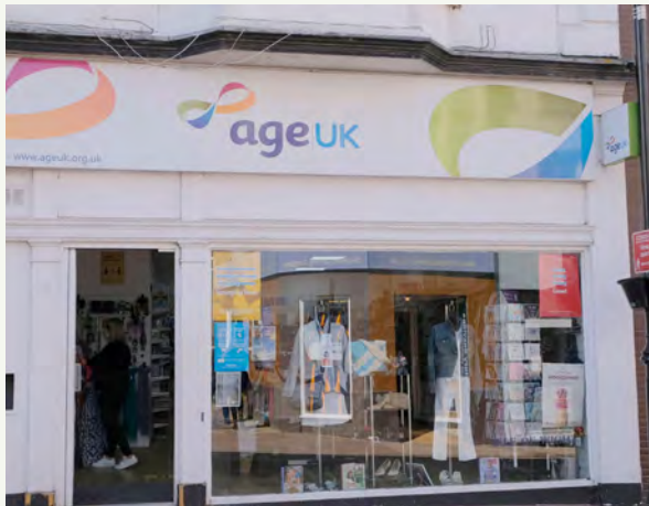
(Left) A poor example of a modern fascia mounted on, and obscuring architectural detail of heritage value. (Right) An example of an additional horizontal, timber batten supported by vertical post and used to achieve an angled fascia.
