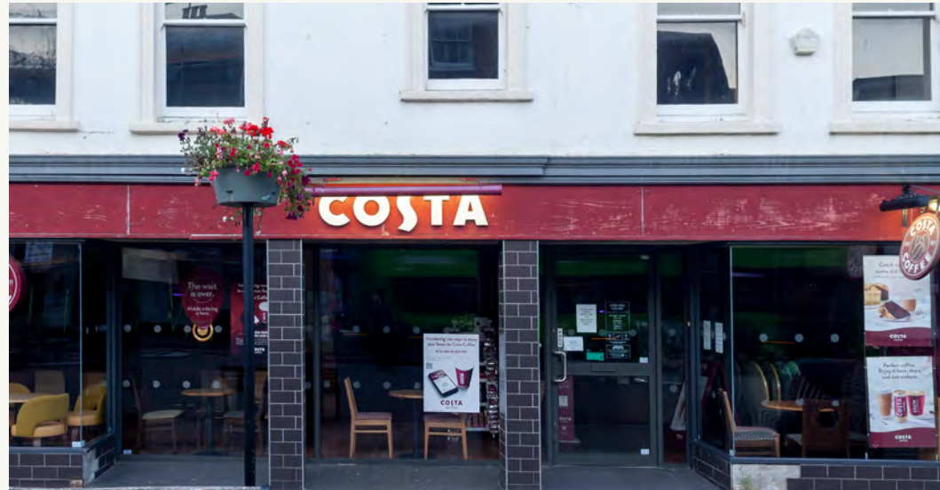
This Costa Coffee is an example of a poorly retrofitted shopfront onto a non-standard commercial frontage which used to be a local inn.
