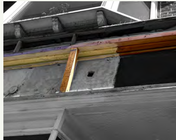
(Left) A poor example of a modern fascia mounted on, and obscuring architectural detail of heritage value. (Right) An example of an additional horizontal, timber batten supported by vertical post and used to achieve an angled fascia.
