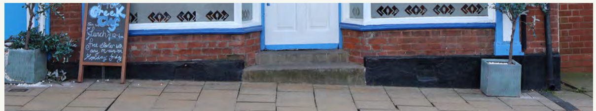
Examples of panelled and brick stallrisers in Lichfield
