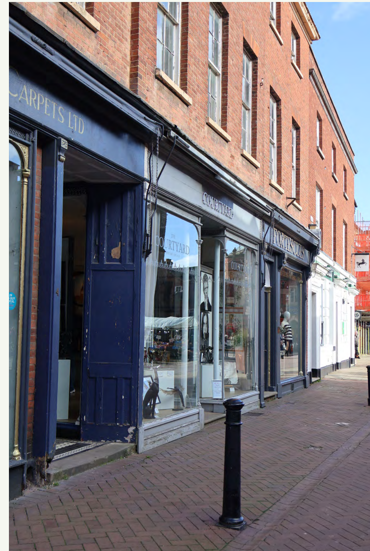
Well designed fascias sit within the corbelling and are proportionate to other shopfront elements.
