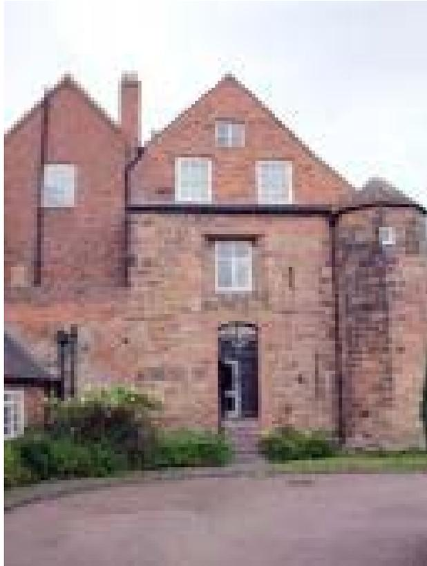
Picture 14.12 Remains of sandstone, fortified walls incorporated into St Mary's House
