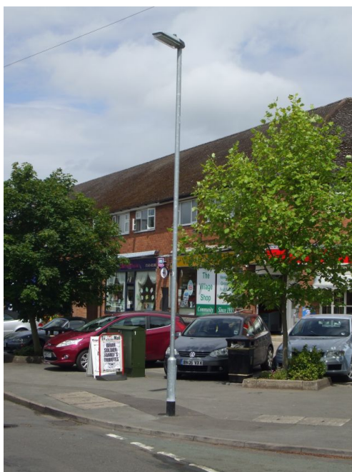
Picture 11.1 Galvanised steel lamp post on Main St.
