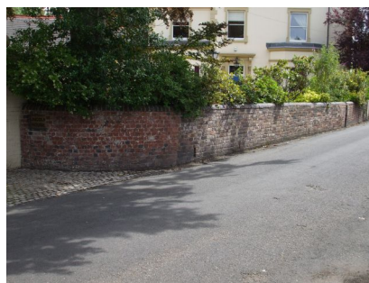
Picture 2.2 Boundary wall, Lincoln House.
