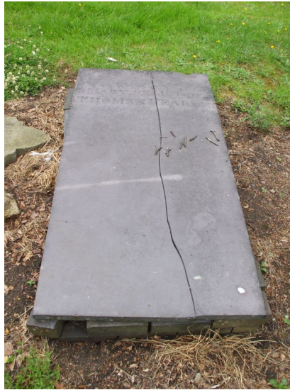
Picture 8.6 Damaged tombstone, St John's Churchyard.
