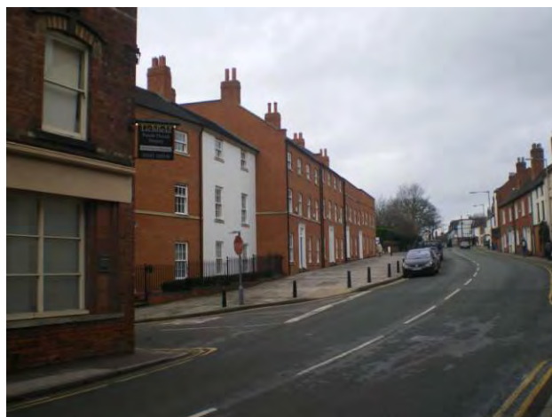
Plate 33: Early 21st century redevelopment on Beacon Street
