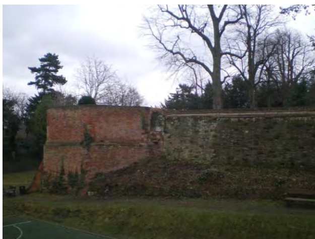
Plate 24: Moat and boundary wall
